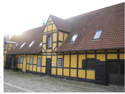
The half-timbered building is 45 bays long and nine bays deep. The bays are remarkably small, around 1,1 m. The roof is clad in tiles and has a fall of around 50 degrees. Two lift dormers rise noticeably above the facade. The building is primarily orientated towards the courtyard due to the original function.
