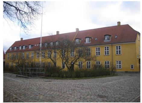
The building is 18 bays long and two storeys high. The roof has a high pitch, in which the four chimneys and fire parapet stand out, with a half-hipped gable to the south and a standing gable to the north. There are 13 dormers towards the courtyard, 11 towards the street and also a number of skylights that provide light to a utilized roof storey. The plinth of the building is very low and one can therefore enter almost directly into the building.
