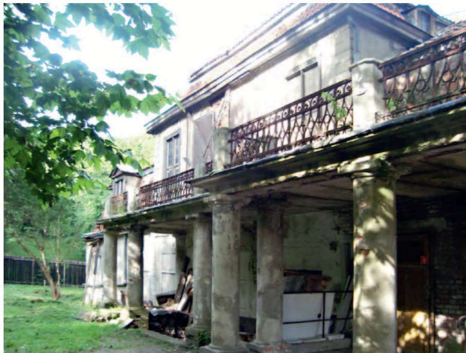
Manor house before refurbishment, Studzienka, Gdansk, Poland
