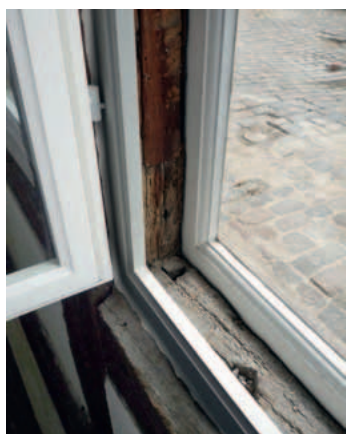
Faestnings Materialgard – Secondary glazing frames, Copenhagen, Denmark
