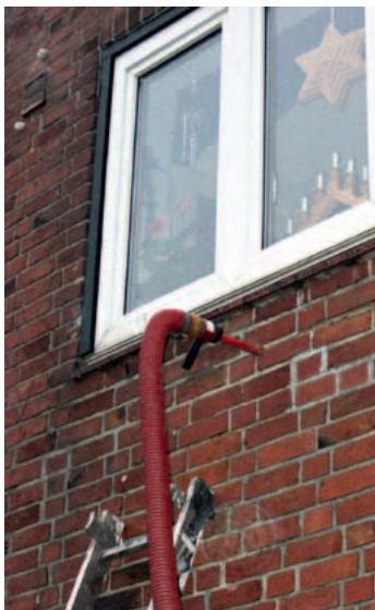
Cavity wall insulation, Kiel, Germany
