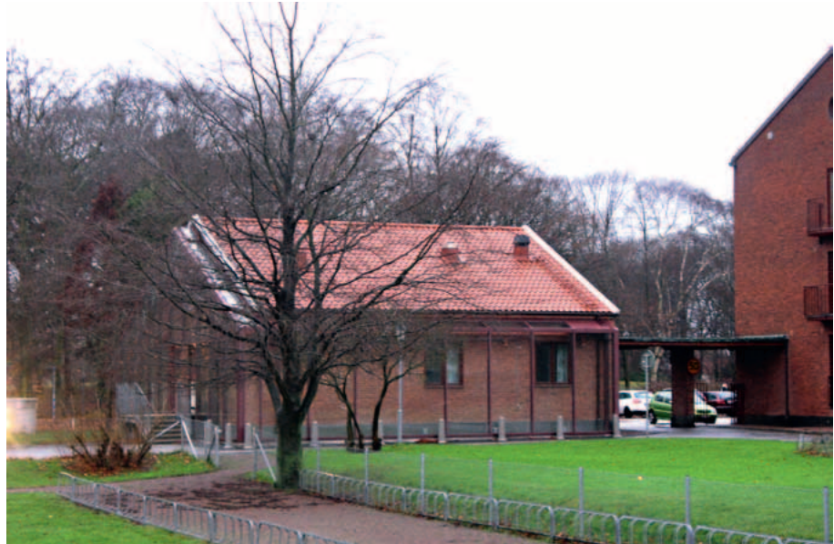
Former gatehouse, Sege Park, Malmö, Sweden
