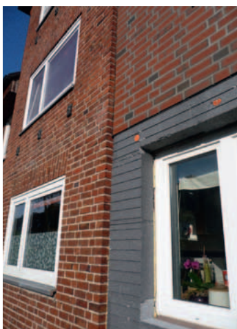
External wall insulation with brick tiles, Kiel, Germany
