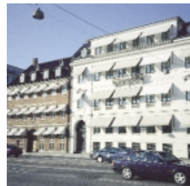
Retrofit: retractable fabric awnings (Source: J Goulding, ERG)
